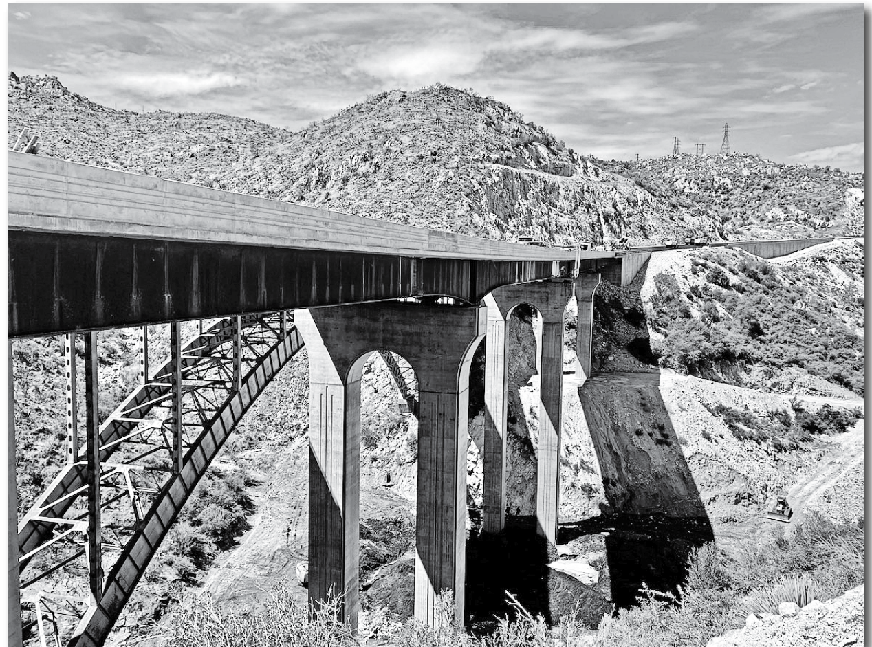
A view of the new bridge over Pinto Creek on U.S. 60 between Superior and Miami. You can see the 72-year-old bridge behind it. ADOT | Submitted
