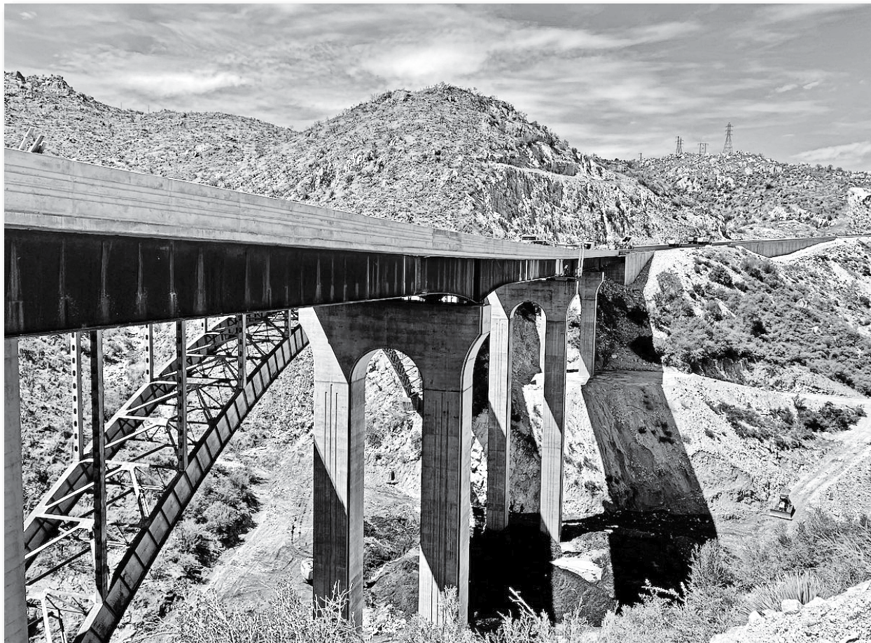
A view of the new bridge over Pinto Creek on U.S. 60 between Superior and Miami. You can see the 72-year-old bridge behind it. ADOT | Submitted
