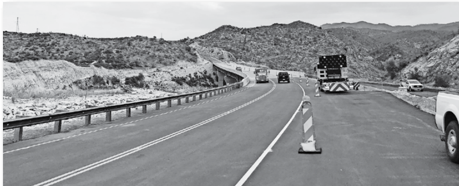
The new Pinto Creek Bridge.
