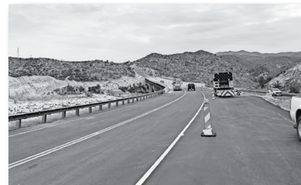
Pinto Creek Bridge now open for traffic.
