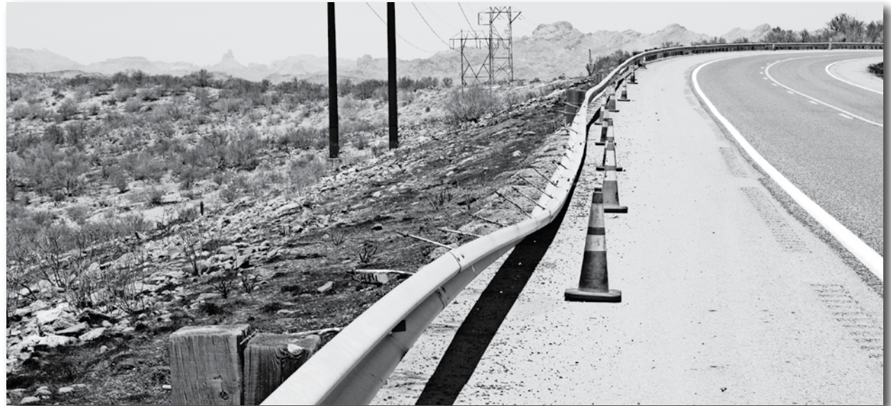
Drivers should be extra careful when Arizona Department of Transportation workers are replacing burned and damaged guardrails. James Carnes | CBN
