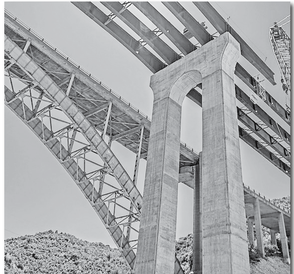
Pinto Creek Bridge, the old and the new, side by side.
