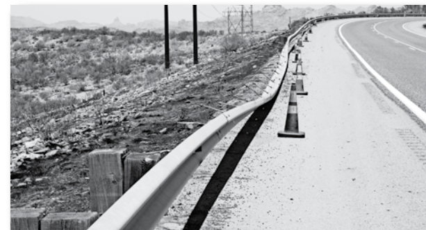
The guard rail posts were burned in several places on Hwy. 177 between Kearny and Superior.
