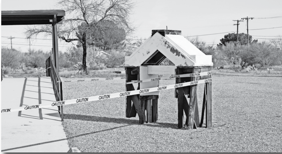
The old bell tower is removed.
