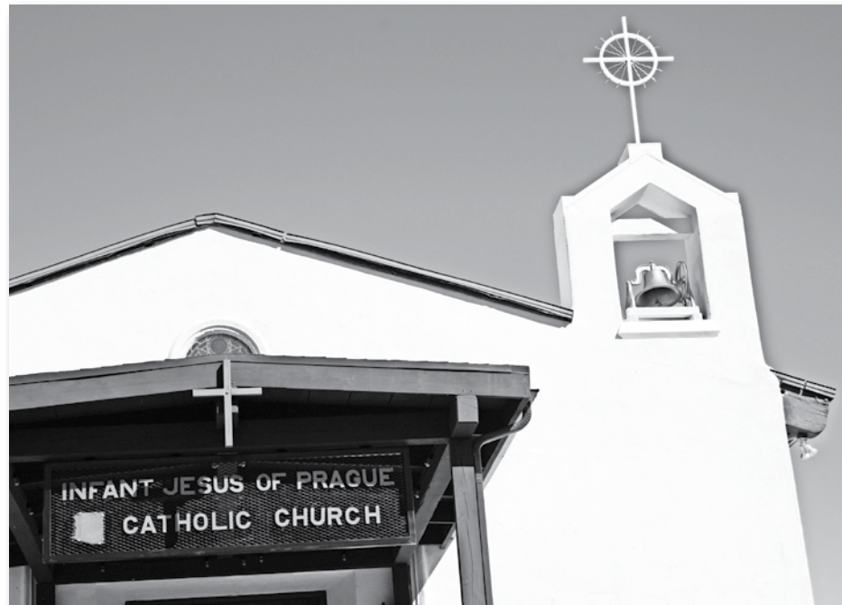
The new bell tower is in place on the church.
