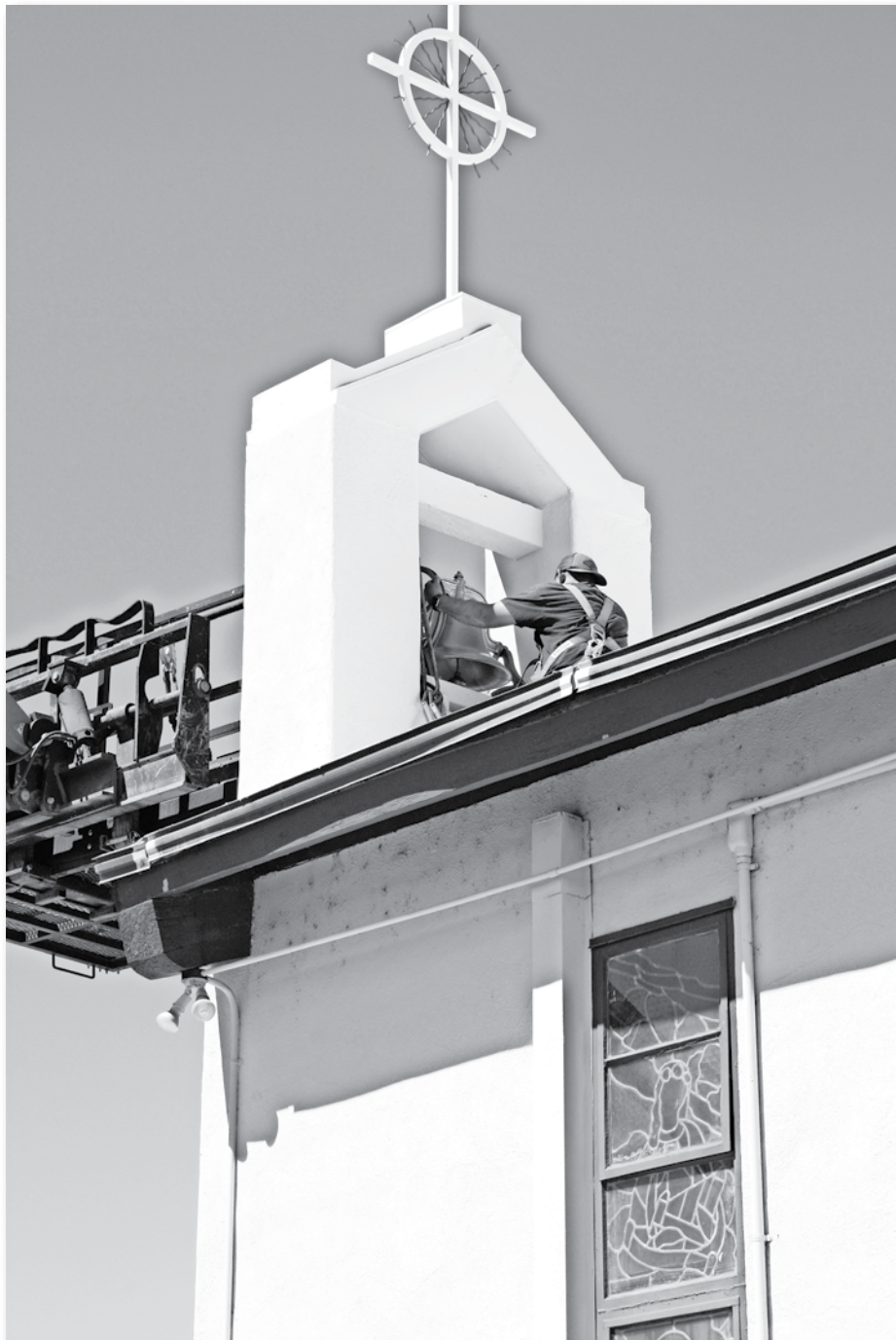
Installing the bell.
