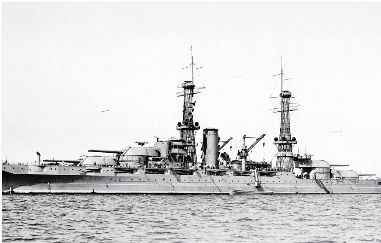
A port view of the U.S.S. Arizona c. 1930.
