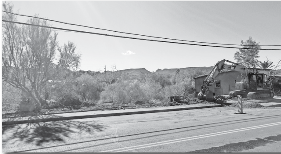
Demolition completed at 679 Main St.
